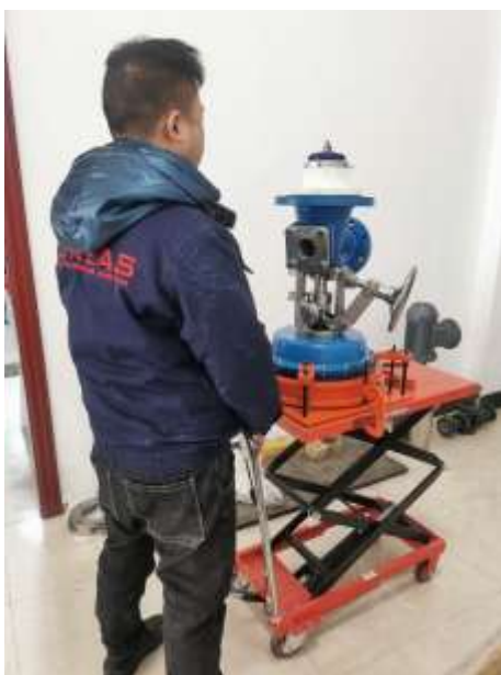
Vertical lift For Bottom Discharge Valve installation 出料閥安裝垂直升降車
